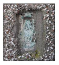
On the side wall of the building known as the Commercial Bar, you can see an Ordnance Survey flush bracket – sadly no longer needed for measuring heights above sea level. This one is number G1977.
